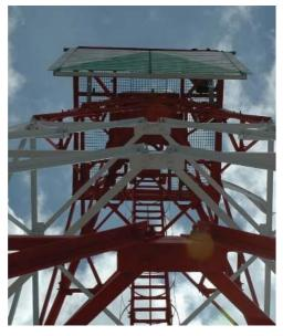
Mediterraneo's Steel Towers model MTS have been especially designed to integrate long-range rotating beacons c/w their solar power supply system.
